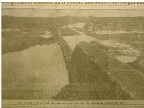
(a) The Picone levee (see Fig. 7) after the 1926 flood (from La Gazzetta di Puglia, 1926).
