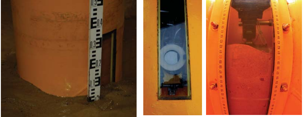
Fig. 1: Photos of the observation window at the monopile and of the installed camera (left hand and middle photo from outside of monopile) and recorded sand level in the scour (right hand side from inside of the monopile).
