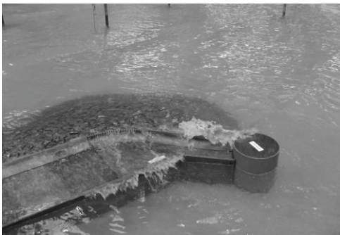
Figure 2. Wave Attack on the Existing Albert Quay
