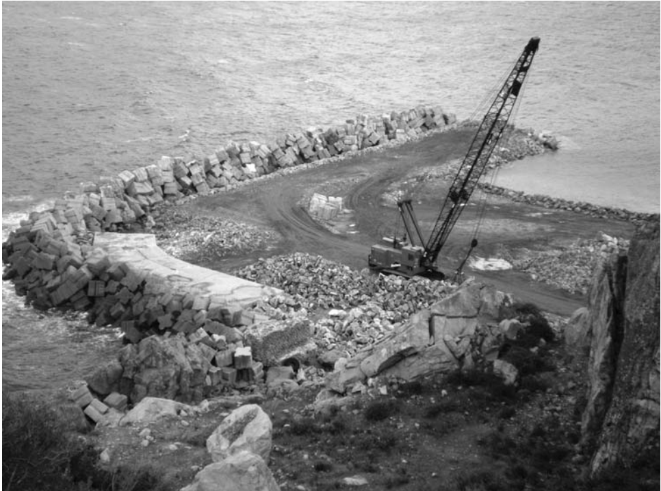
Figure 7: Harbour Construction Work Underway
