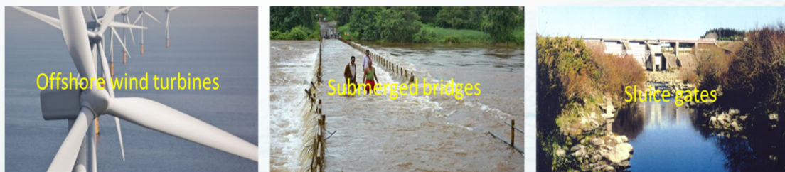
Figure 1. Three cases of scour at hydraulic structures.
