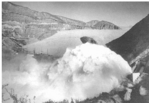
Figure 1. Trajectory spillway at Serre-Ponçon dam, France (La Houille Blanche 2 1993, p. 224).
