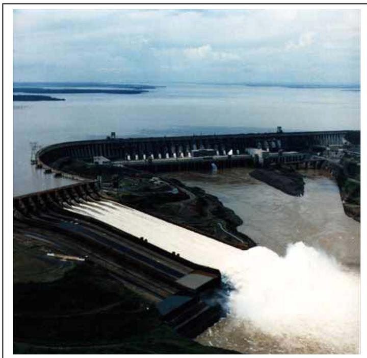
*Fig. 1. A spectacular hydraulic jump at the end of a spillway (by eFluids.com gallery).*
